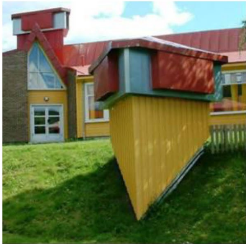
Figure 2.12: ETAHE's intake tower of Mediã school (Paolo and Roberto, 2009).
